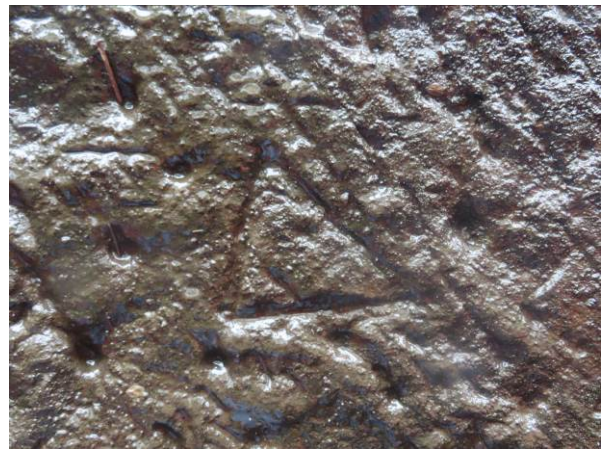
Mason's marks on the stones in the lock walls. Each mason had their own mark, and the marks signified the blocks produced by a particular mason so they could be paid for them.
