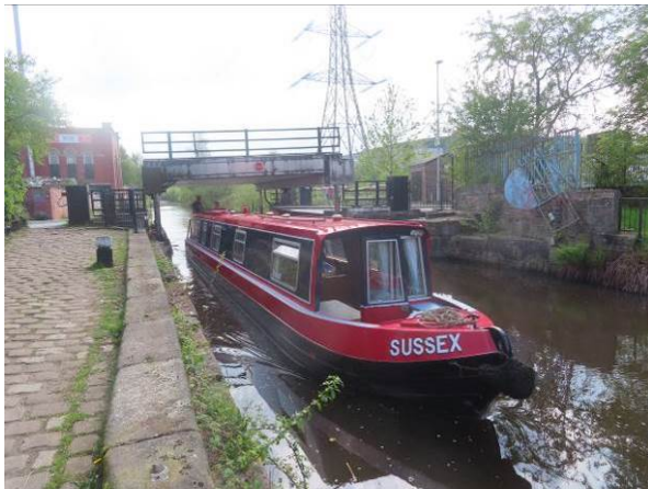
Two projects built as part of the canal's restoration. Left is the Bridge 76a the vertical lift bridge, this bridge was built as part of the canal's restoration and is fully automatic, you turn up, put in a key and push a button and the barriers come down and up goes the bridge.
