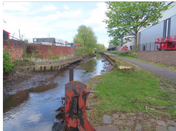
Heading up through East Manchester. The mechanism in the foreground is used to assist in pulling on lock gates with short balance beams.
