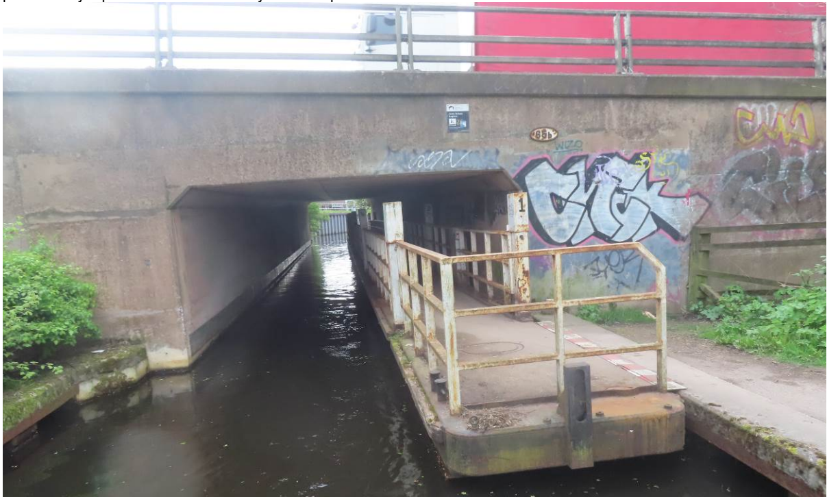
During the canal's closure the M62 motorway was built across the canal, fortunately about 100m east of the blocked canal was an underpass. With a relocation of a lock, it was possible to divert the canal through the culvert. It's a bit narrow for the broad canal, so in order to get the broad boats through the towpath is on a floating pontoon that has to be towed out.
