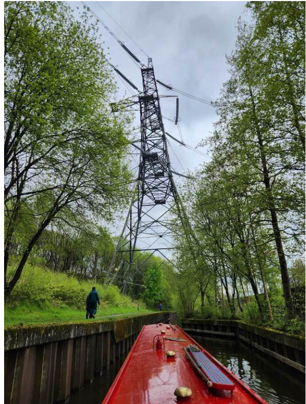
Just west of Scout the canal had been filled in and a pylon built over the canal. When restored a channel was cut through between the pylon's legs.
