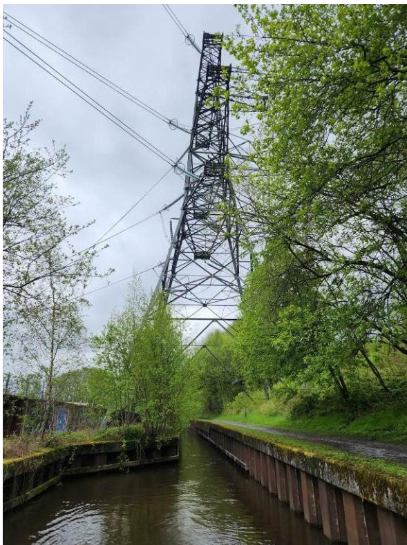
Just west of Scout the canal had been filled in and a pylon built over the canal. When restored a channel was cut through between the pylon's legs.
