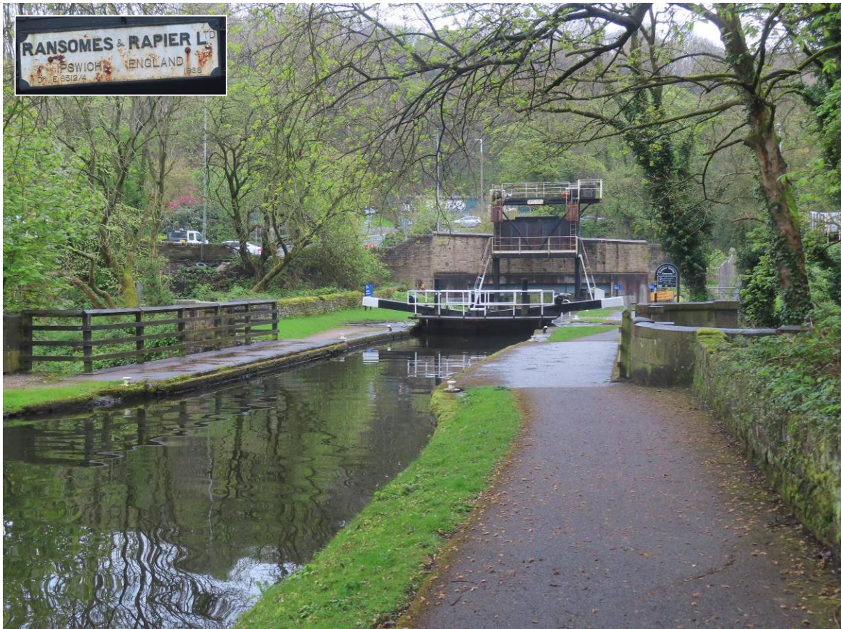
In the 1930's the road across the bottom of the Salterhebble Bottom Lock was widened necessitating the installation of a guillotine bottom gate, this gate moves electrically, rather slowly, and still proudly has a plate saying it was built in 1938.
