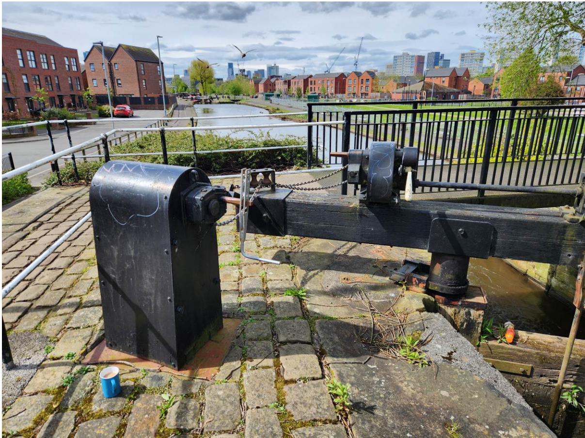
Heading up through East Manchester. The mechanism in the foreground is used to assist in pulling on lock gates with short balance beams.
